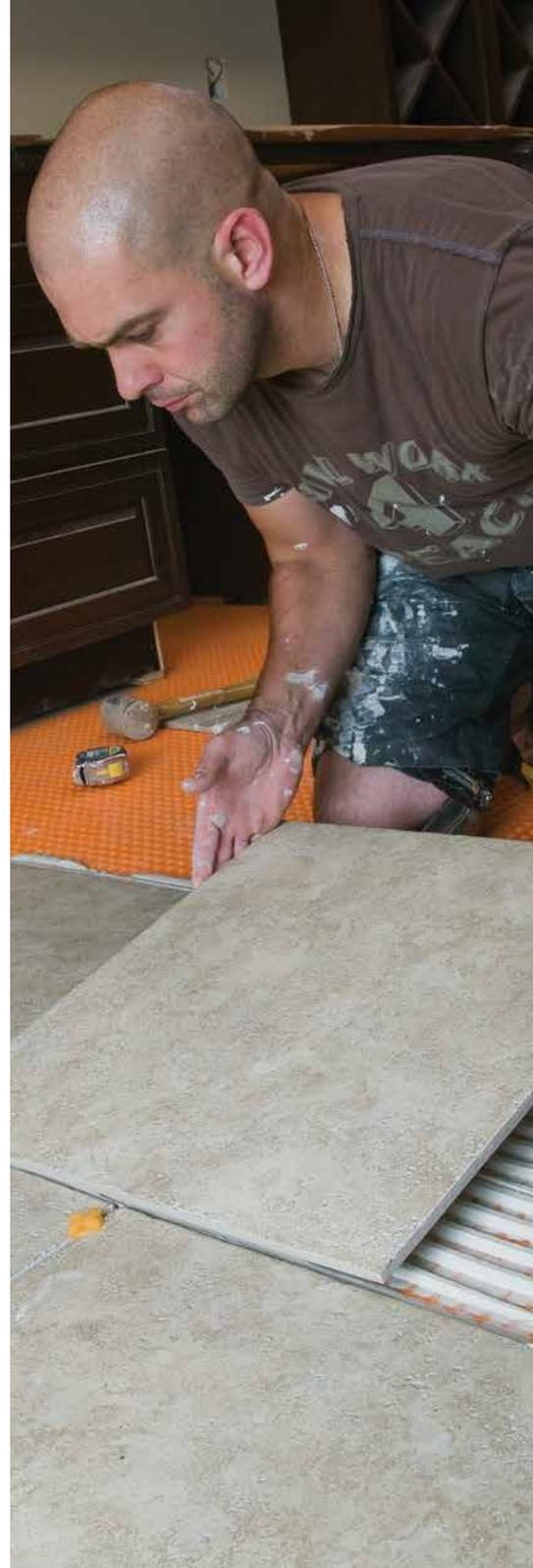
immediately before bedding it firmly into the fresh ribbed adhesive bed with a slight twisting motion to ensure a solid bed and prevent voids under the tile. Some “solid bedding” trowels and pourable adhesives are available that allow the floor tile to be solidly bedded without the need to butter the back of the tiles.
